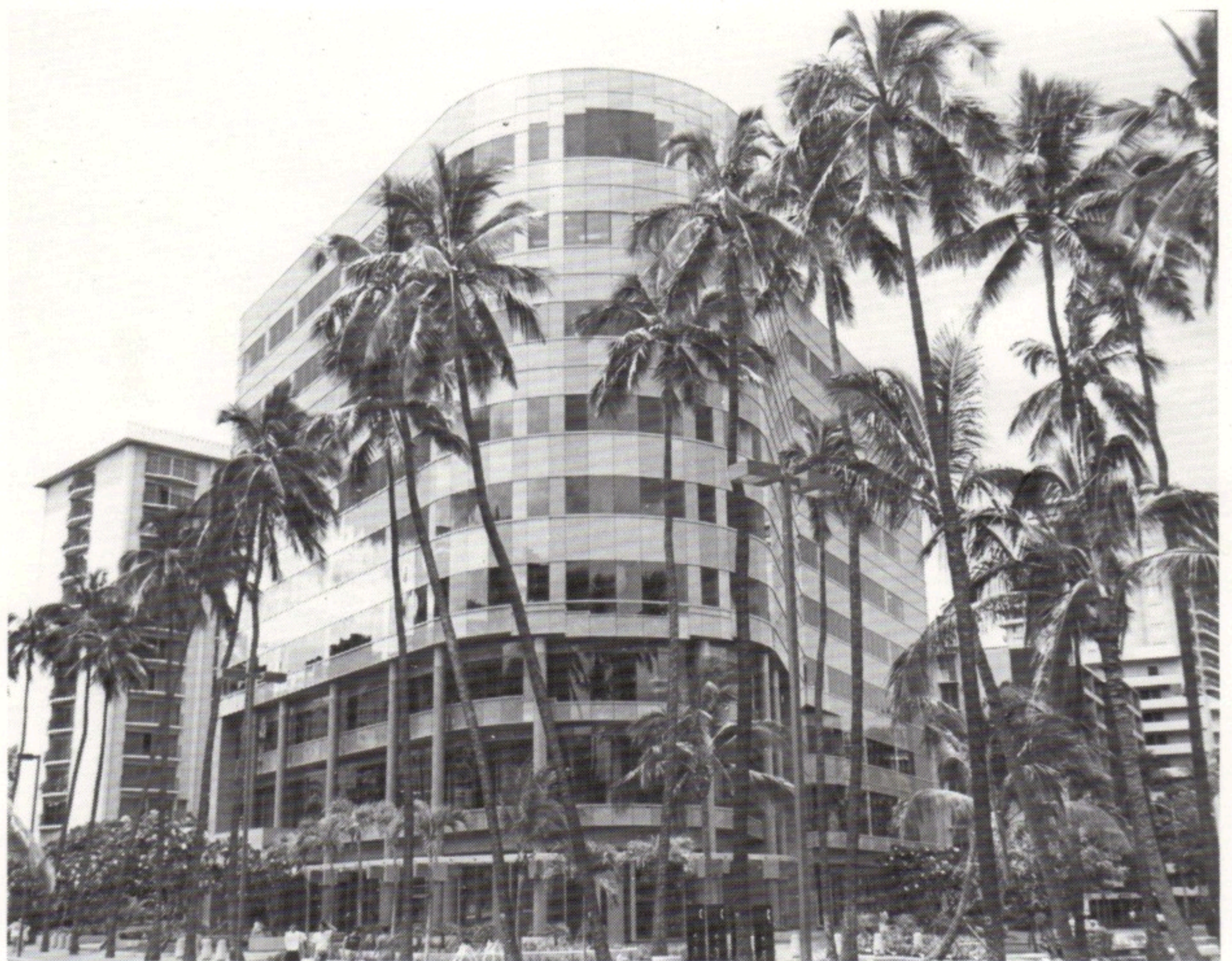
Kalakaua Center under renovation.
