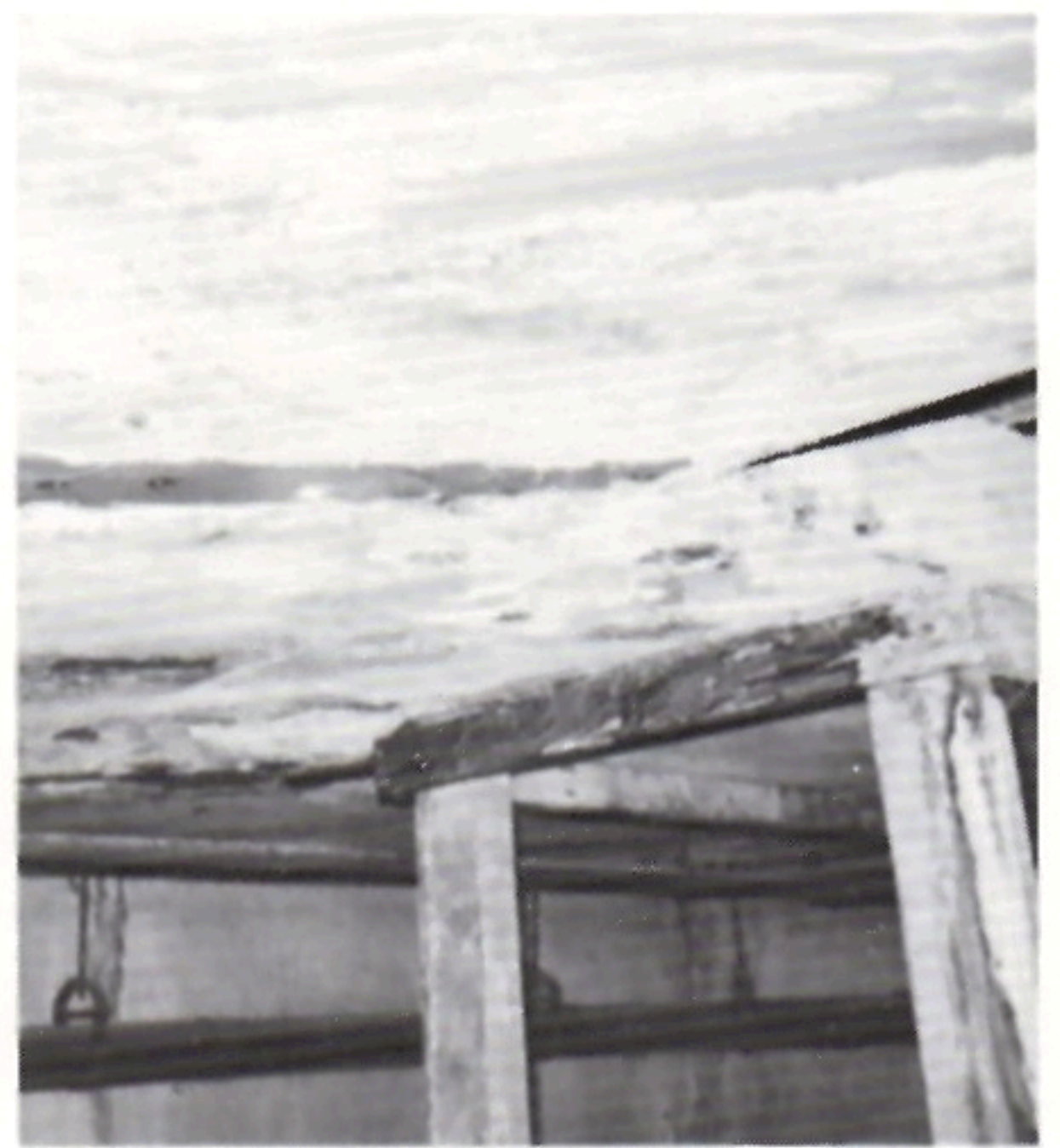
Above, epoxy injection around an earth-filled cavity. Below, the underside of an earth-filled cavity, looking up at a gunite slab.
